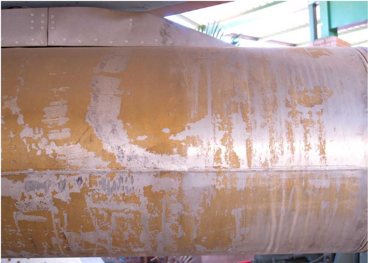
Details of 500 liter RP18R fuel tank showing orange protective coating and distinct tank longitudinal and circumferential weld seams.
