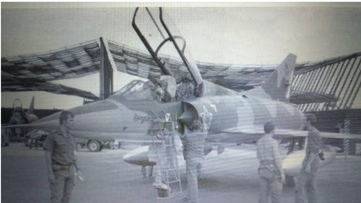
Unidentified BZ on the Border, likely to be Ondangwa. BZ is painted in the early hard edge gloss camouflage with full markings including orange/white/blue rudder and 2 Squadron badge. Natural metal 1,300 liter RP62 wing tanks are installed. The aircraft in the background is a CZ.
