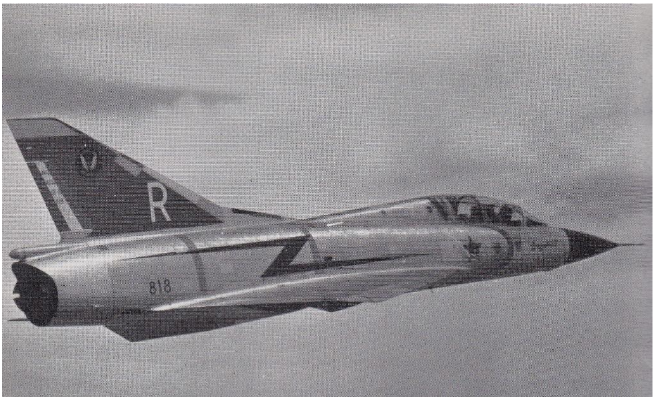
Two images of unpainted natural metal BZ #818 (white R) in the delivery livery. The airbrakes are open and the yellow edging is clearly visible. Note the red trim on the wing leading edge at the fuselage junction. There is no red trim behind the rear cockpit.
